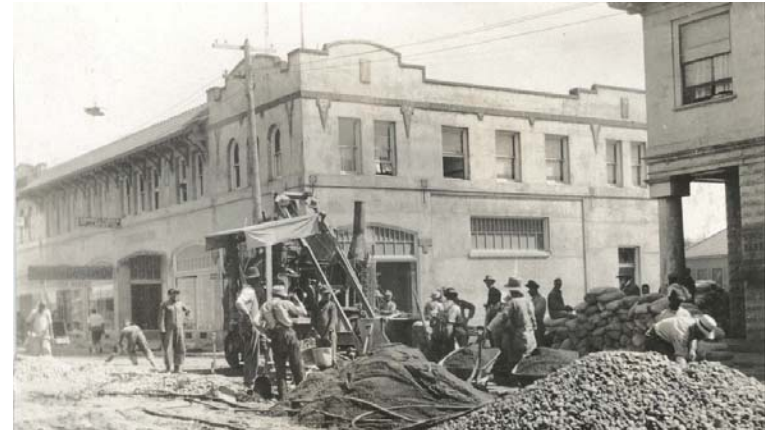
GRADING MAIN STREET AT 4TH AVENUE, 1917
